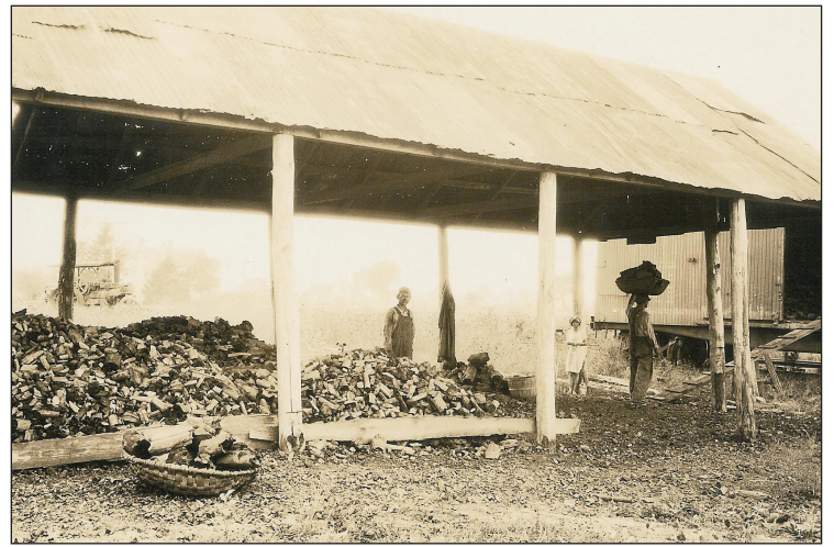
CHARCOAL PRODUCTION: Someone who made charcoal was known as a “collier.” Charcoal was used as a filtering agent for making rum and whiskey, but it was also key to the development of the iron industry. Large ironmaking operations required as many as 400 bushels of charcoal to make one ton of wrought iron, and it took one acre of woodland for 800 bushels of charcoal. These photos show a family operation in Sussex County in 1929. Six cords of pine wood was stacked, covered with pine needles, and then six inches of moist earth. A basket of coal was fed in daily through a hole in the top. The fire burned for several days with a few holes to allow gas to escape.
