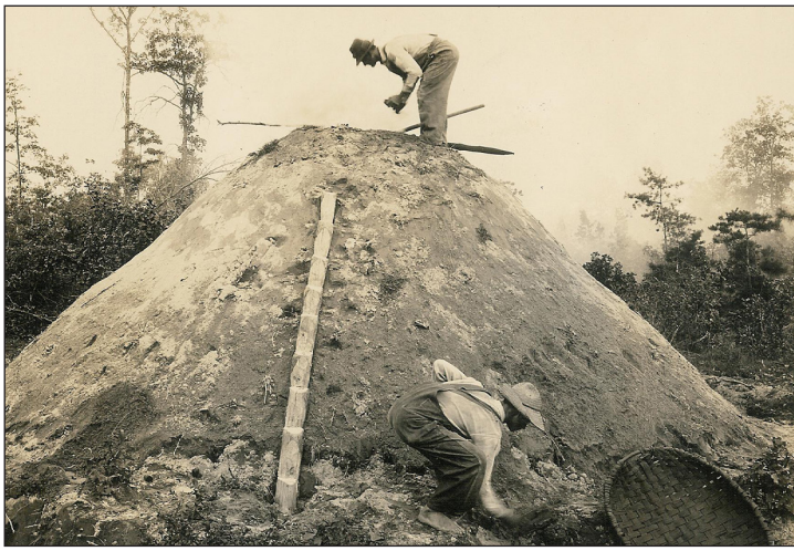
CHARCOAL PRODUCTION: Someone who made charcoal was known as a “collier.” Charcoal was used as a filtering agent for making rum and whiskey, but it was also key to the development of the iron industry. Large ironmaking operations required as many as 400 bushels of charcoal to make one ton of wrought iron, and it took one acre of woodland for 800 bushels of charcoal. These photos show a family operation in Sussex County in 1929. Six cords of pine wood was stacked, covered with pine needles, and then six inches of moist earth. A basket of coal was fed in daily through a hole in the top. The fire burned for several days with a few holes to allow gas to escape.
