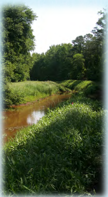
Tax ditch in Sussex County
